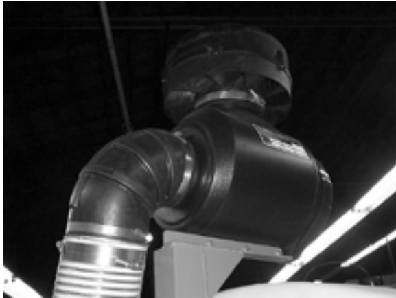
Air filter assembly P/N 7870 With pre-cleaner P/N 8244
